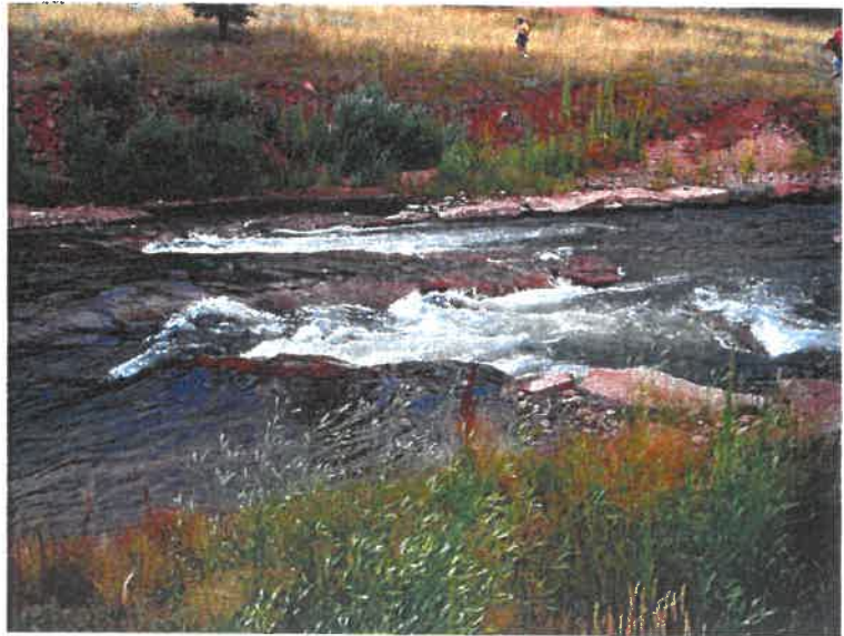
Figure 4: W-weir installation in Colorado at low flow.
